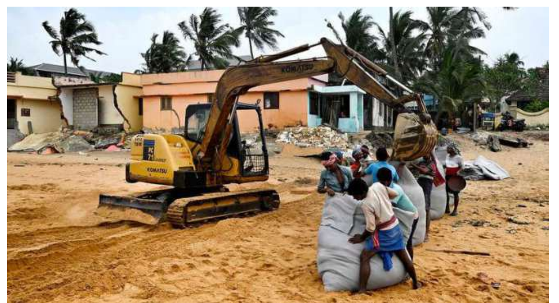
On a war footing: Workers prepare sandbags as protection against high tidal waves on the Shanghumugham beach in Thiruvananthapuram. NIRMAL HARINDRAN
